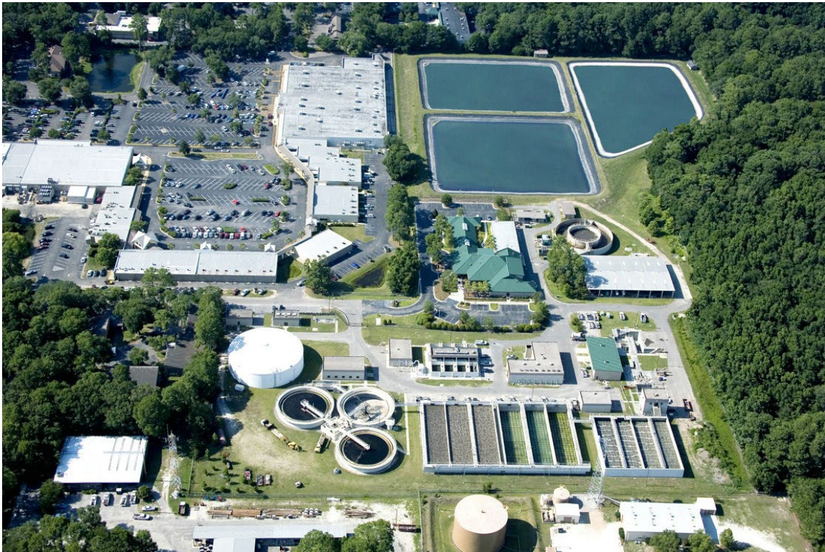
The PSD Customer Service Center and Recycled Water Plant
