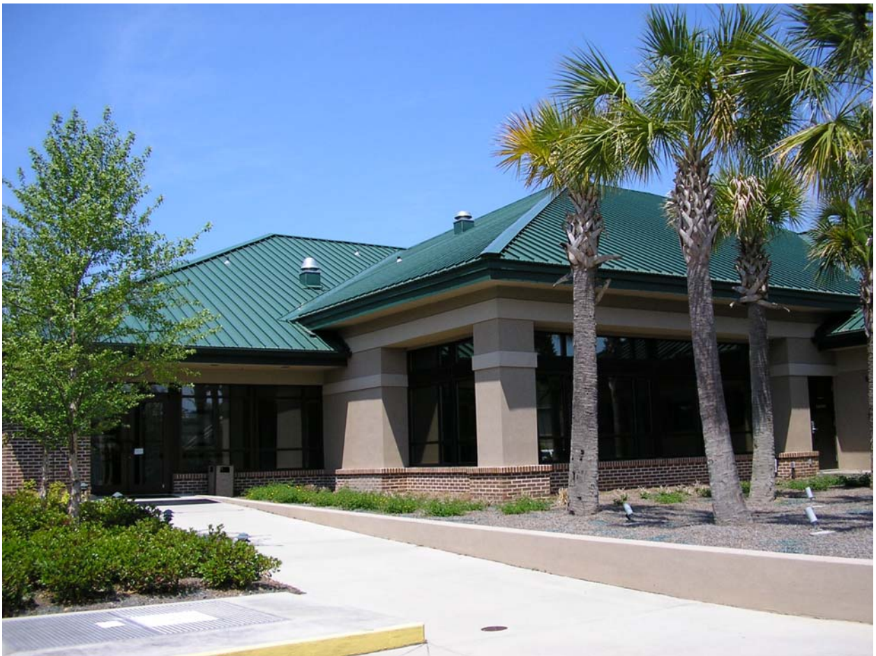
The Hilton Head PSD Water Resources Center, 21 Oak Park Drive, Hilton Head Island, SC
