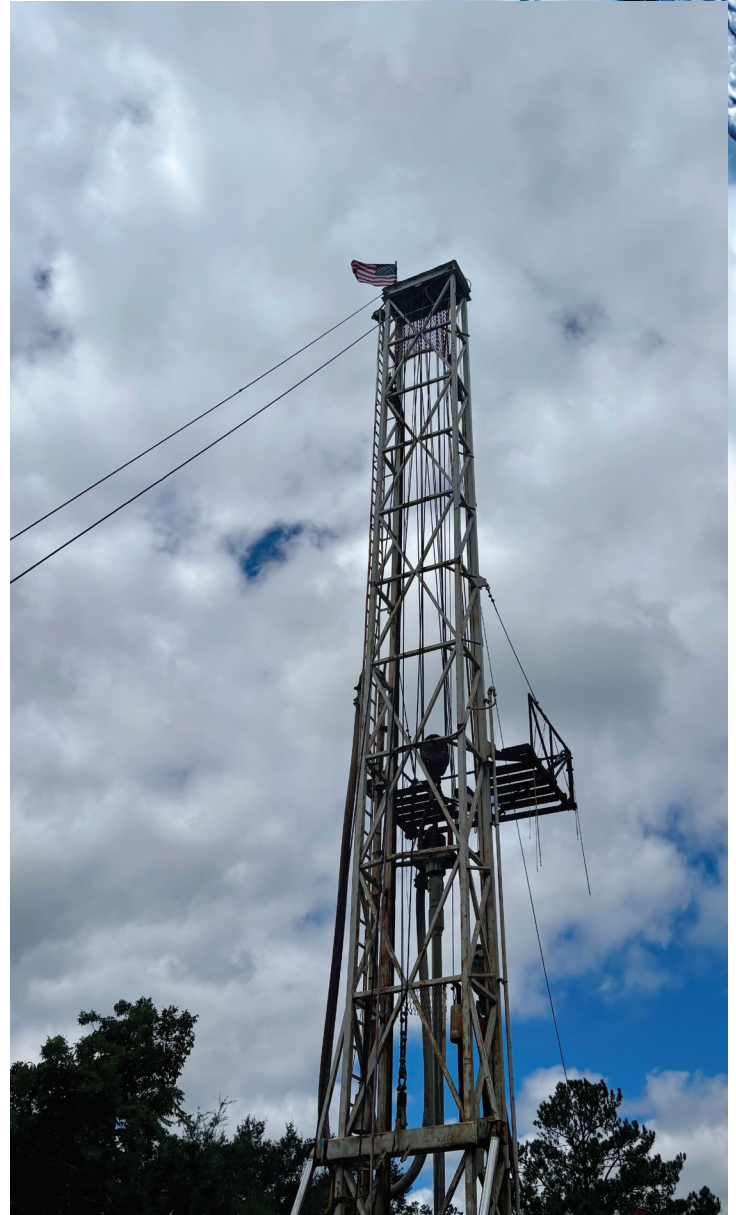
The drill rig for the deep well at the Old Welcome Center location
