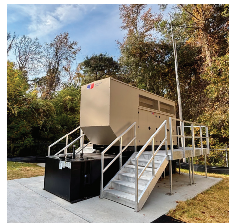
Generator for the new Booster Pumping Station
