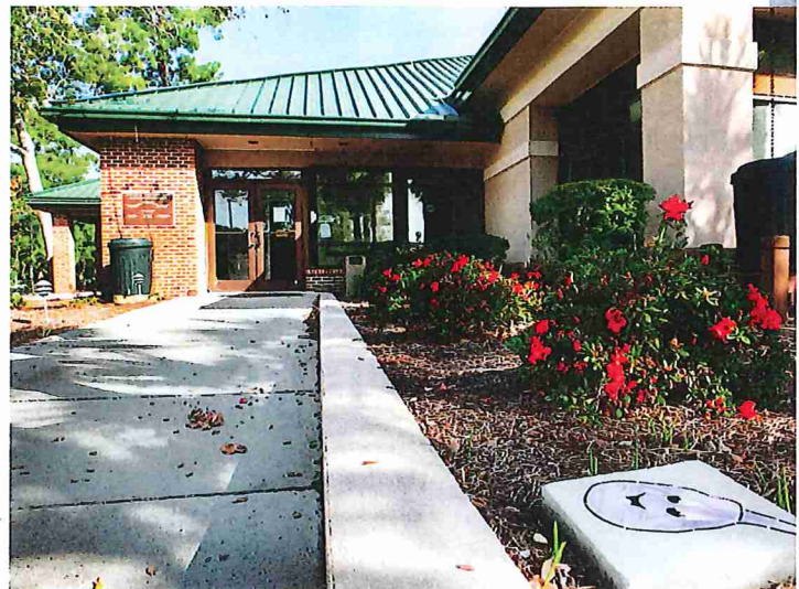
The headquarters of the Hilton Head Public Service District. The wastewater treatment plant has 6.4 mgd design capacity.
