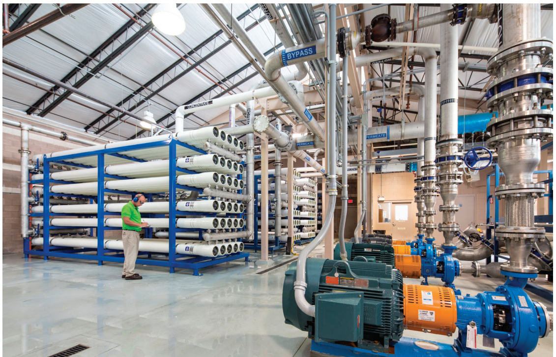
Jim Hewitt, the PSD's Operations Superintendent, checks the new filters at the utility's Reverse Osmosis (RO) Water Treatment Facility. The facility has been expanded to provide 4 million gallons of fresh water a day.
