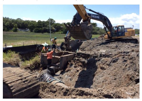
A crew works on the relocation of the PSD's 24-inch water transmission pipeline in greater Bluffton.
