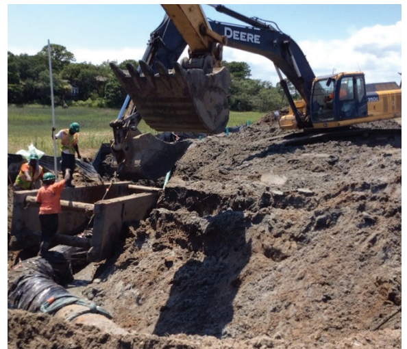
A portion of the PSD's water transmission pipeline that supplies wholesale water from the mainland was relocated as part of the Bluffton Fly-Over project. About 30 percent of the PSD's water supply comes from wholesale water.
