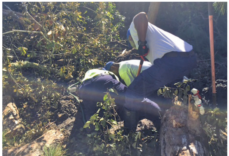
PSD first responders Doug Nice, Andre Swinton, and James Washington work to repair a broken water connection in the Bear Island area in Hilton Head Plantation during the recovery from Hurricane Matthew.
