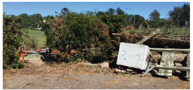
The storm toppled trees that smashed the PSD's sewer pump stations at Headlands (top) and Old Fort in Hilton Head Plantation.
