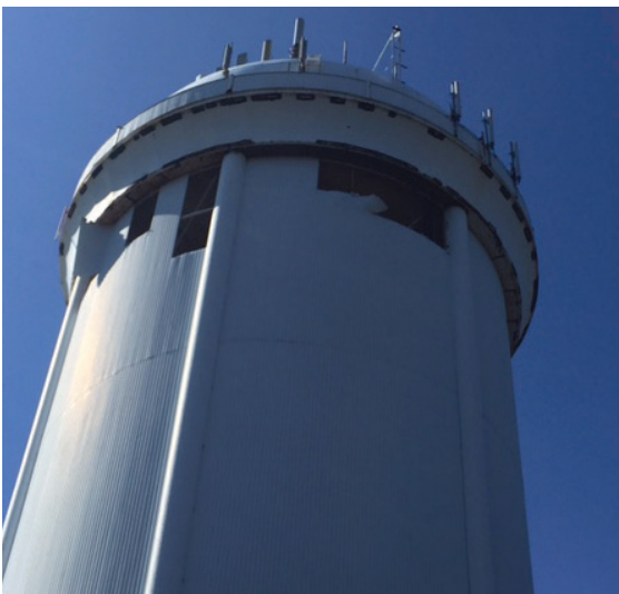
Hurricane Matthew tore the metal skirting from the top of the Union Cemetery Water Tower and deposited it on the ground below.
