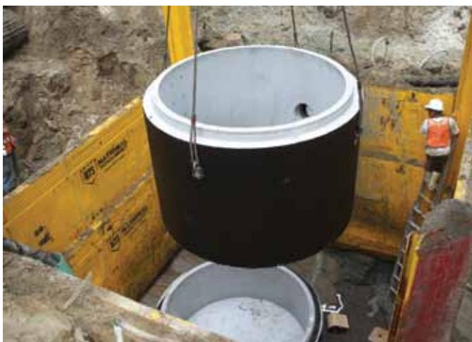
The PSD constructed a sewer pump station to serve the mid-Spanish Wells Road area.
