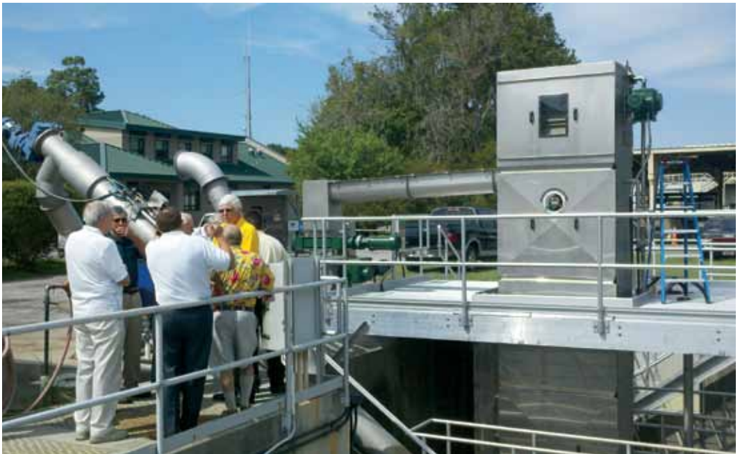
The “Muffin Monster” is a state-of-the-art machine that removes large solids from the wastewater stream and makes our treatment process more efficient.
