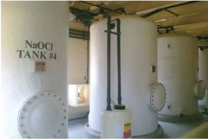
The PSD uses sodium hypochlorite – or liquid chlorine – to treat recycled water.
